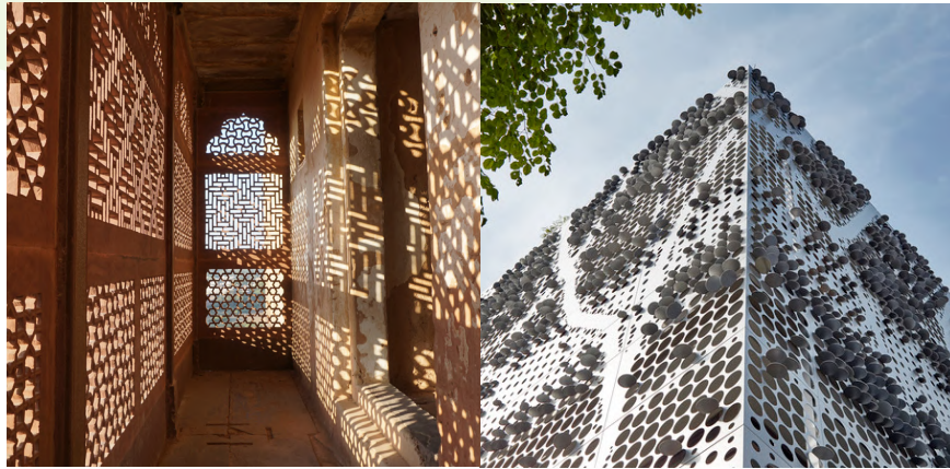
Above: (Left) Low-tech Jaali solutions used in traditional houses in India and (Right) High-tech building facade system by WOW Architects in Camo House, Singapore to deal with thermoregulation.
